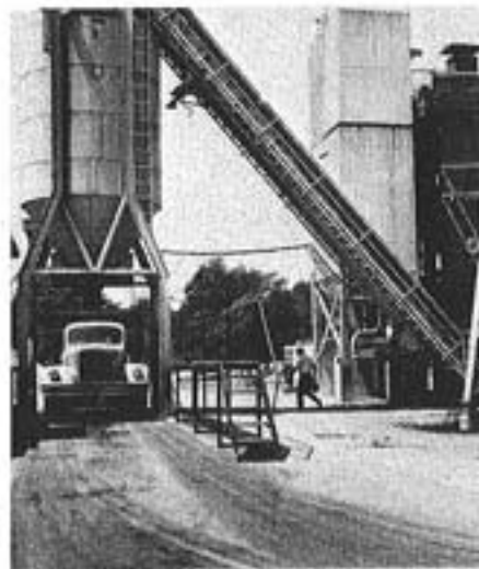
Each truck (left) is loaded with a pre-set tonnage of sand emulsion mix while it stands on scale platform with digital weight control.
